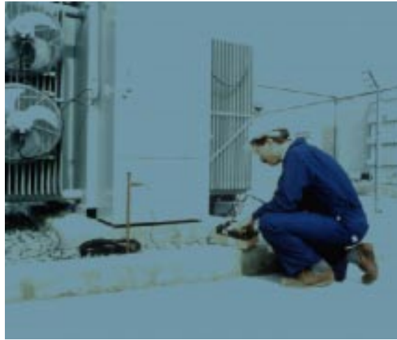
Figure 6-5—Ground resistance testing
